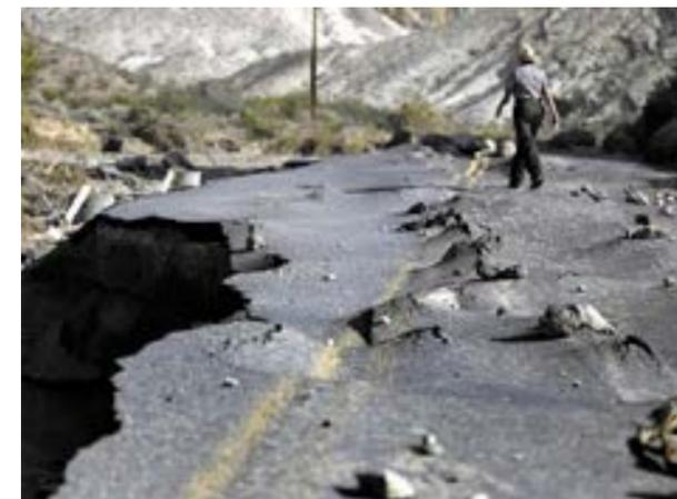
A 100-yard-long section of newly paved Highway 267 in Grapevine Canyon, a two-lane road designed to withstand severe flooding, was lifted up by roiling water and then slammed down on boulders in Death Valley National Park. (Brian van der Brug / *Los Angeles Times*)
